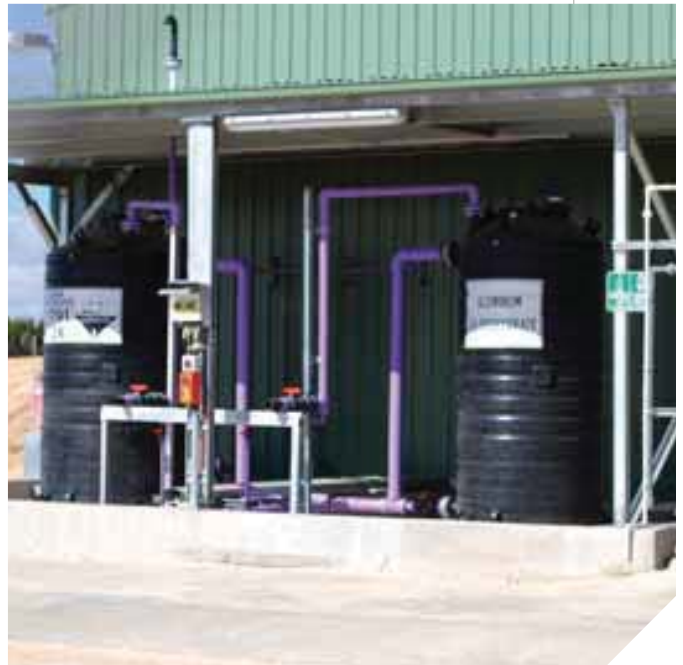
Water treatment plant, South Australia
