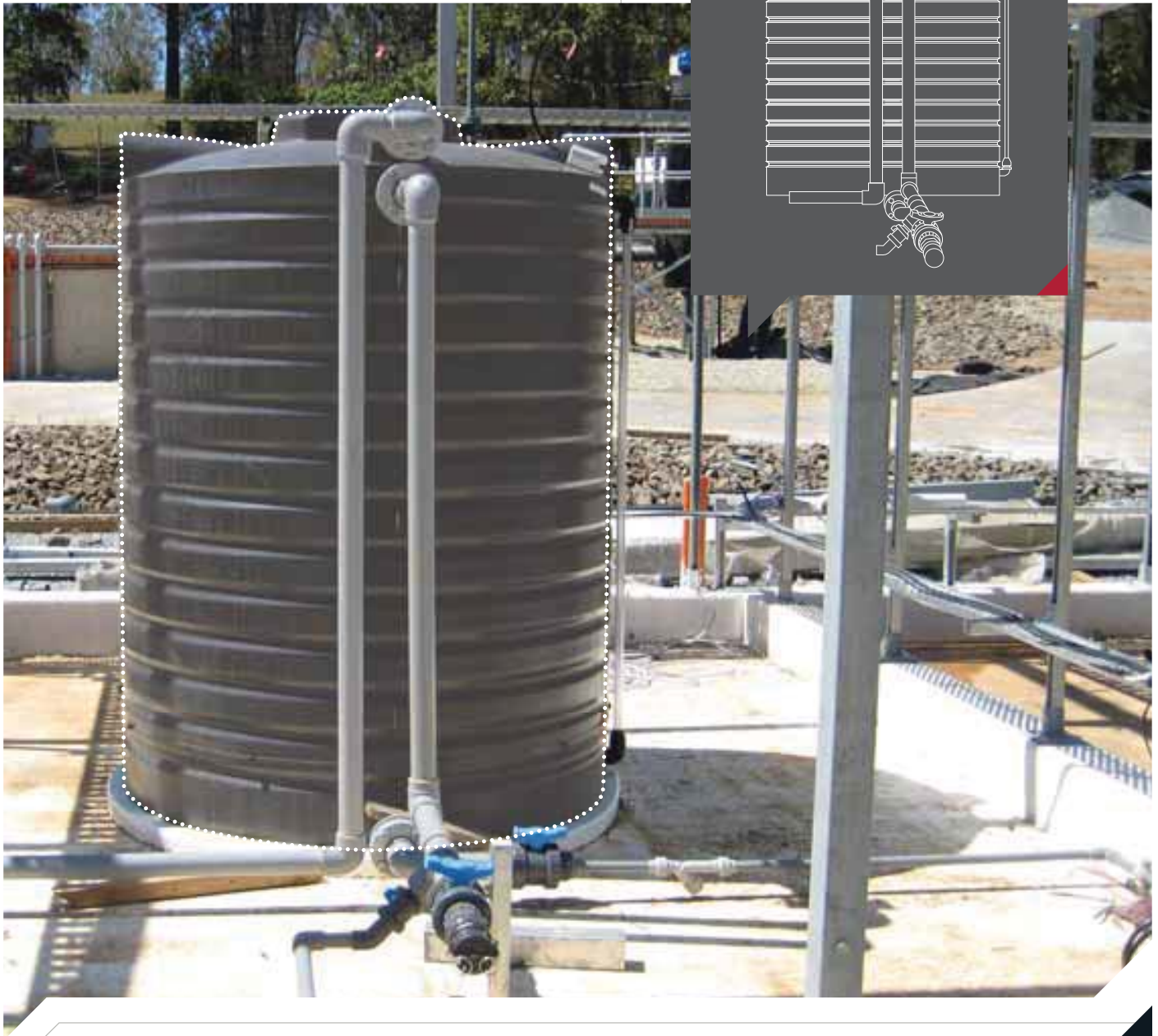
Dosing tank at a water treatment plant
