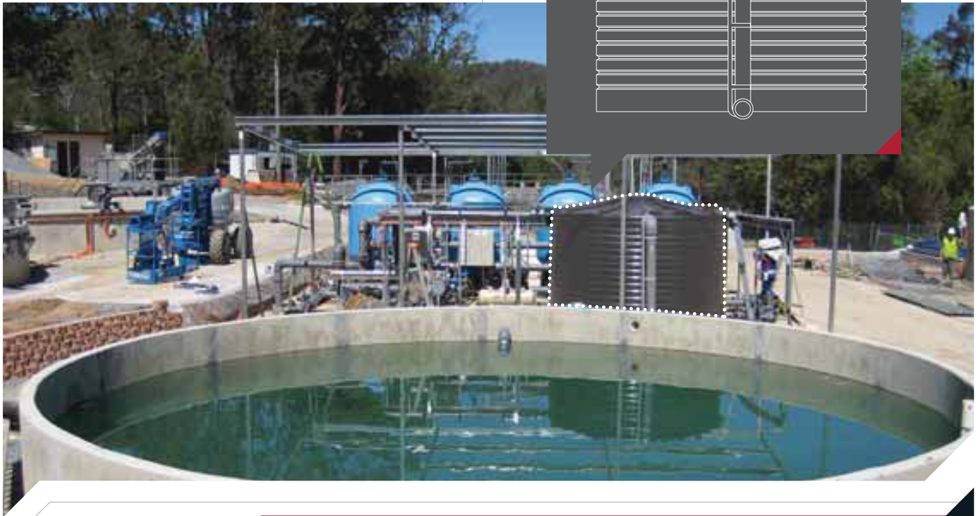
Effluent treatment plant, Gold Coast
